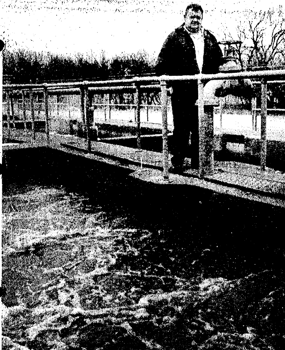
SEWAGE TREATMENT IN PROCESS: Cal Penix, an employee at the Chelsea sewage treatment plant, watches one of the activated sludge tanks in which sewage is kept stirred up and exposed to air so bacteria can work to break it down. Solids settle to the bottom, and the treated liquid is piped into Letts Creek.
